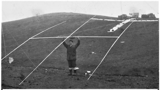
Working on The Beam
